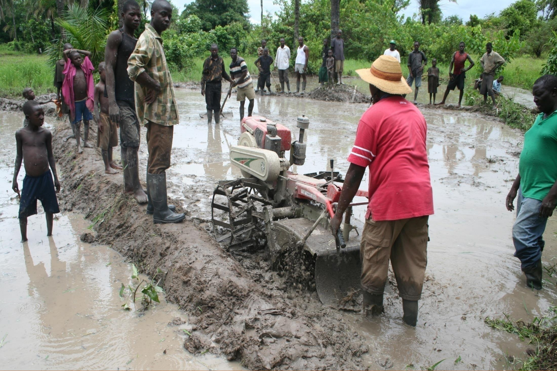
Sawah Development at Shabamaliki village, Bida, Nigeria.
